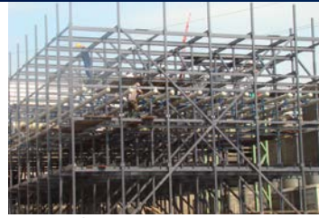
FRP cooling towers – construction phase
