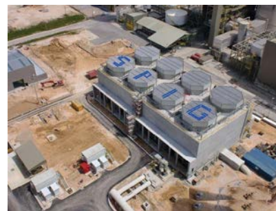
Noise-abated cooling towers at an 800 MW power plant
