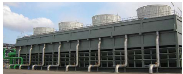
Concrete cooling towers
