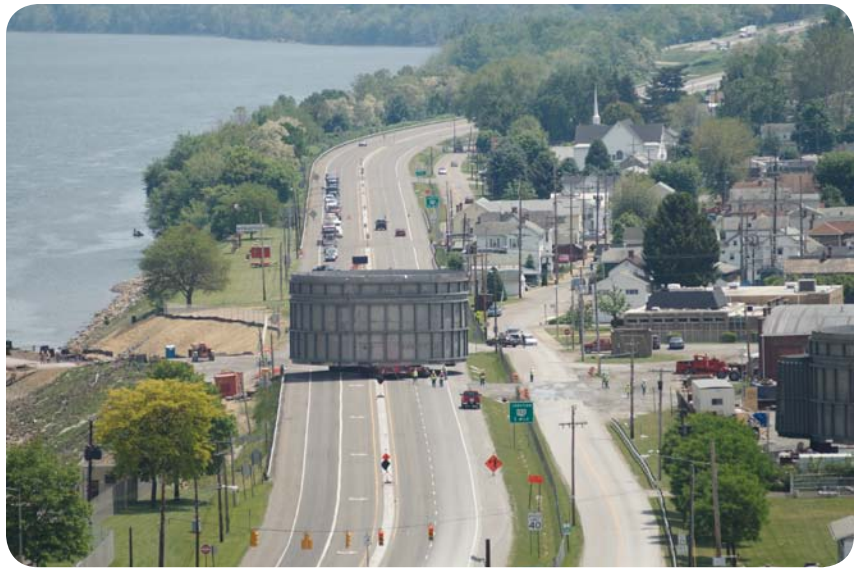
Wet FGD module crossing highway from barge unloading.
