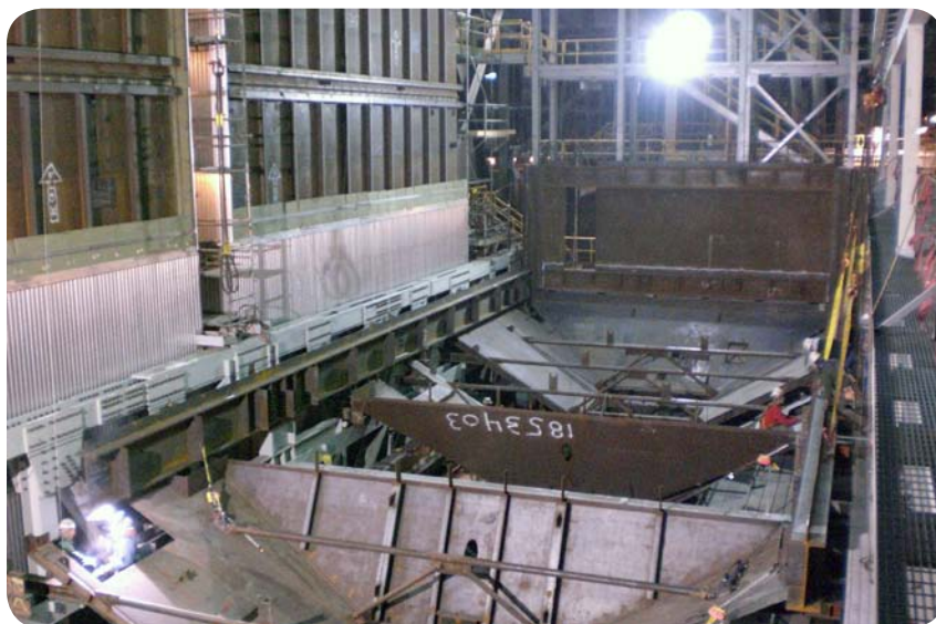
Unit 6 SCR reactor under construction.
