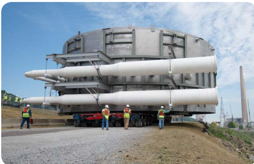
Wet FGD module on transporter moving to plant for installation.
