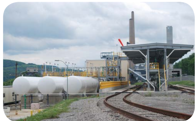
Ammonia storage tanks and rail station, along with the necessary pumps, valves and piping were all part of BWCC's balance of plant responsibilities.
