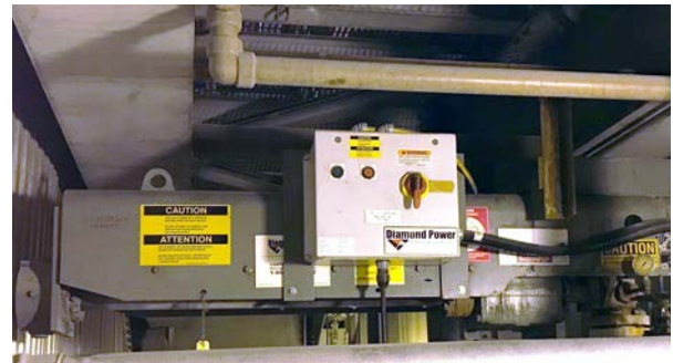
B&W's Diamond Power IK-700-AH retractable sootblowers feature complete coverage in timing with the rotational speed of the air heater for improved cleaning
