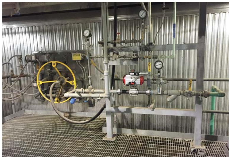
The Diamond Power HydroJet water cleaning system with associated valves and plumbing assembly features a compact design for easy access.
