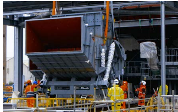
DynaDischarger ash extractor being positioned under the grate.
