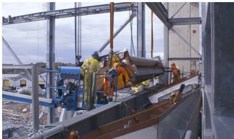
One of the ten modular DynaGrate sections being lifted into place.
