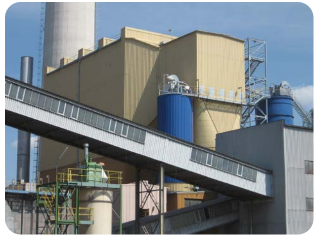
A CDS is ideal for plant locations with limited space because of its smaller footprint.
