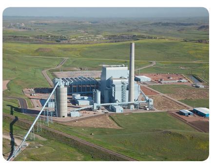
The 400 MW Dry Fork Station features a RB Carolina-type pulverized coalfired boiler and B&W AireJet<sup>®</sup> low NO<sub>x</sub> burner technology.
