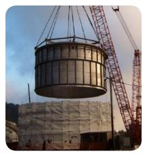
The construction plan included an on-site scrubber module fabrication area that produced absorber modules for both the Fort Martin and Hatfield's Ferry sites. This plan optimized modularization opportunities because off-site modularization was not feasible due to access constraints created by locks on the adjacent Monongahela River.
