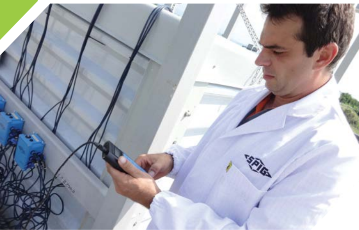
Continuous monitoring with the UNICO system provides plant personnel with important real-time operating data, enabling them to make performance-enhancing operational decisions.
