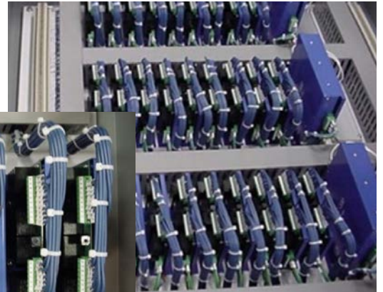
Typical PRC-100® rapper control cabinet
