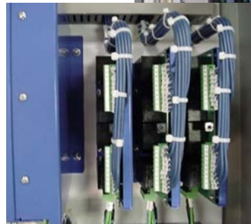
Typical PRC-100® rapper control cabinet
