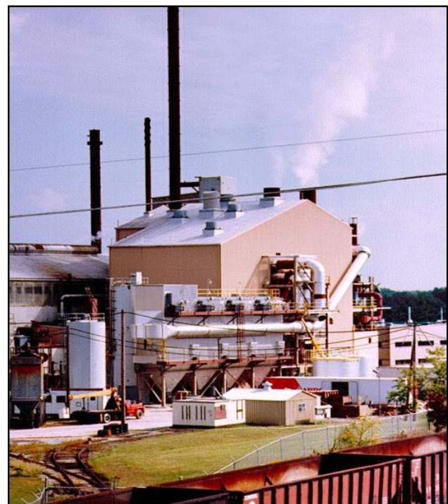
Fig. 2 B&W PGG's Clean Environment Development Facility (CEDF).
