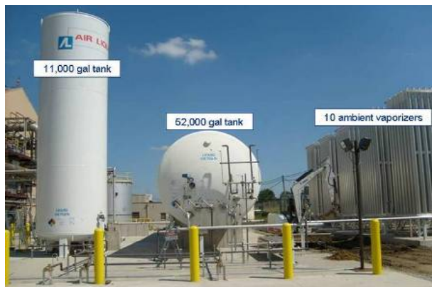
Fig. 5 Oxygen supply system.
