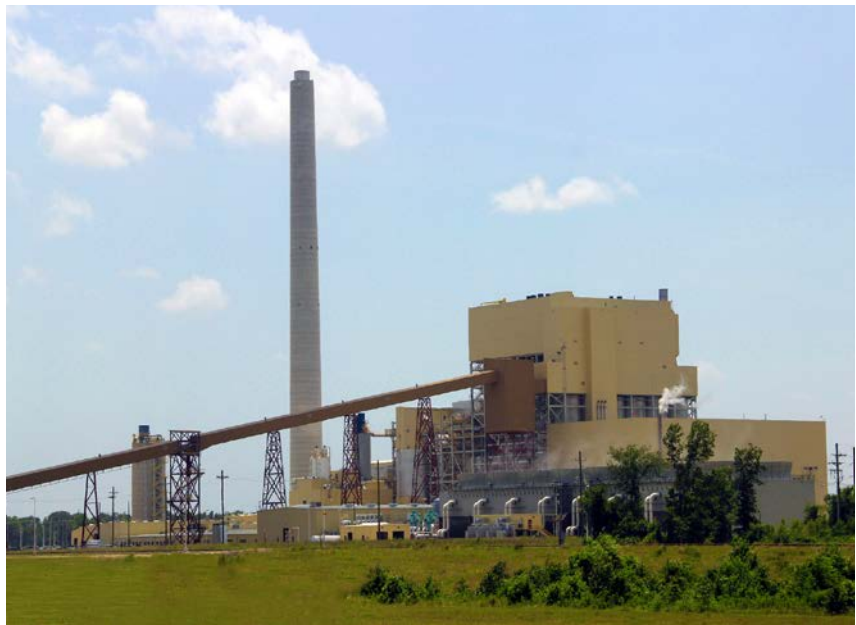
The 600 MW John W. Turk, Jr. Power Plant features ultra-supercritical boiler clean coal combustion technology and advanced emissions control equipment.
