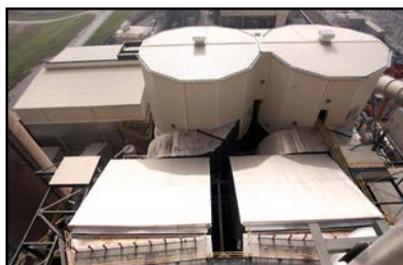
*Pollution control equipment on Hawthorn Unit 5 includes an SCR system for NO<sub>x</sub> reduction, dry FGD for SO<sub>2</sub> control, and a pulse jet fabric filter for particulate control.*
