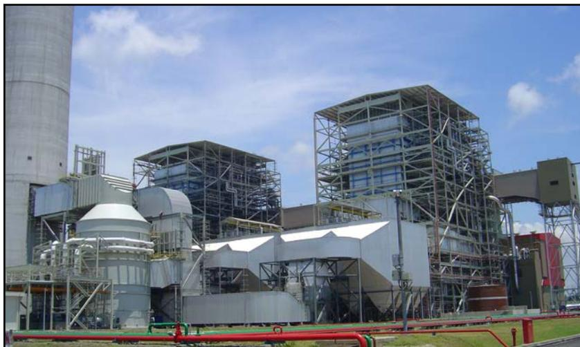
Environmental equipment at the Tanjung Jati power plant includes low NO<sub>x</sub> burners, wet FGD system, and electrostatic precipitators.
