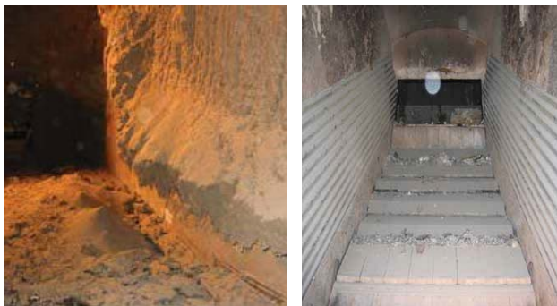
Slag deposits in a furnace with uncooled refractory (left) and the rebuilt plant with water-cooled wear zone (right) after 4000 hours of operation.
