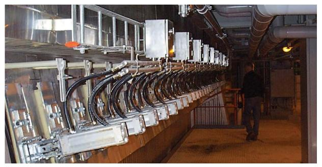
A complete installation of FlexRod port rodders replaces difficult, hot and dangerous manual port cleaning and is ideal for both primary and secondary air levels.
