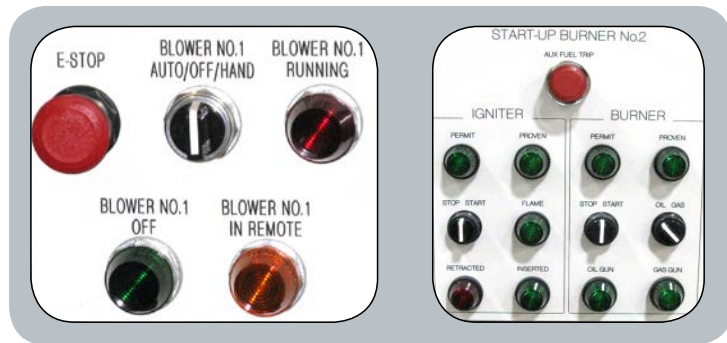
Cooling air blower and igniter burner controls.
