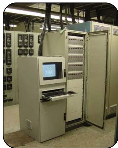
A typical Flame Doctor system installation analyzes individual burner performance for optimum combustion.
