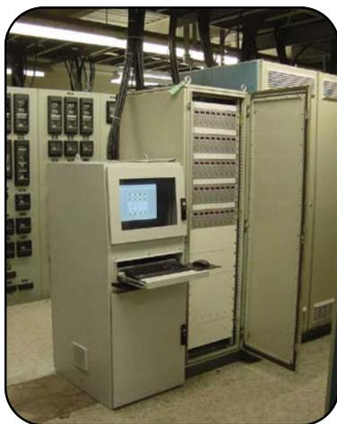
*A typical Flame Doctor system installation analyzes individual burner performance for optimum combustion.*
