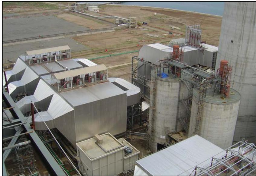
B&W's dry electrostatic precipitator has a proven record of performance and reliability.
