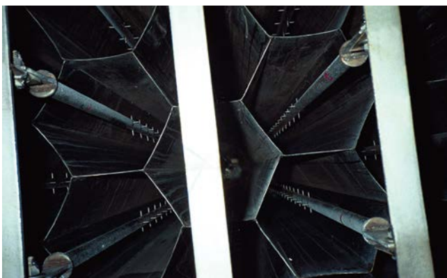
The hexagonal gas passage design allows for a more compact unit configuration and lower pressure drop.
