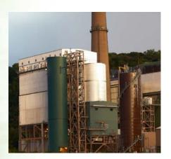
Circulating Dry Scrubber Systems Through an exclusive North American license with Hamon Enviroserv GmbH, B&W provides a circulating dry gas desulfurization technology (also known as a circulating dry scrubber or CDS). CDS technology, designed to reduce SO<sub>2</sub> and other emissions, is ideal for smaller units firing medium to high sulfur coals or for units with site specific needs.
