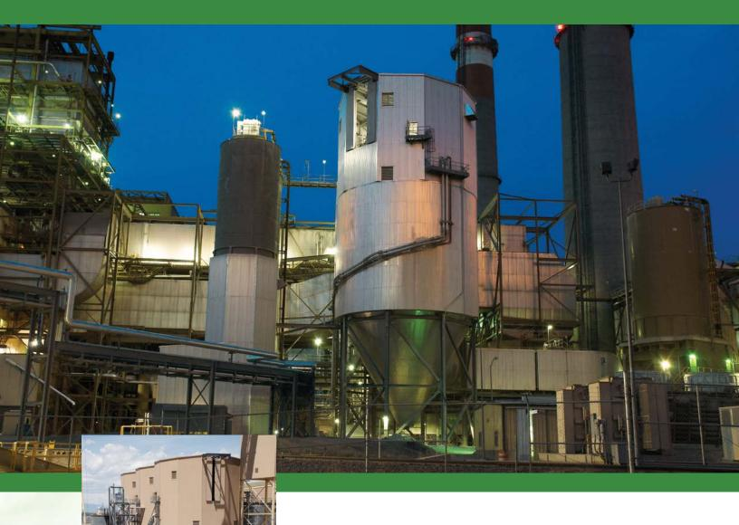
**Spray Dryer Absorber Systems** are licensed by B&W from GEA Process Engineering A/S for the GEA Niro spray dry absorption (SDA) process. Our customers benefit from high SO<sub>2</sub> removal efficiencies, high system availability, low capital costs, and low operation and maintenance costs, as well as the inherent capture of oxidized mercury.
