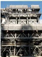
**Dry Electrostatic Precipitators** B&W's particulate control experience began with the first electrostatic precipitator (ESP) installation in the U.S. in 1907. Our dry ESP combines the advantages of maximum collection efficiency and low operating and maintenance costs with extensive application experience. We also provide engineered upgrades, quality components and services to help keep your ESP operating at peak performance levels.
