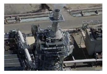
The WGS jet ejector venturi (JEV) technology is an ideal choice for partial-burn units, where the available flue gas pressure is low. The JEV creates suction pressure at the venturi throat from the action of the recirculated scrubber liquid. The application of WGS JEV scrubbing may avoid the need to upgrade older CO boilers. This JEV design offers the lowest required inlet pressure of any commercial scrubber.
