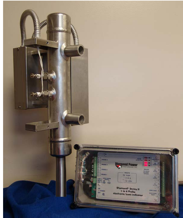
Diamond Power® Series II 1 to 4 Probe ELI with steam/water differentiator
