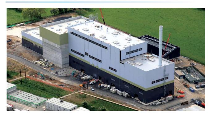
Located some 40 kilometres north of Dublin, Ireland's first waste-to-energy plant began delivering electricity to the city's grid in November 2011. Babcock & Wilcox Renewable (B&W) provided the boiler, combustion grate, combustion control, and selective non-catalytic reduction (SNCR) system.
