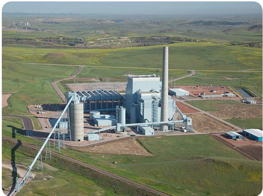
*The 400 MW Dry Fork Station features a RB Carolina-type pulverized coal-fired boiler and B&W AireJet® low NO<sub>x</sub> burner technology.*
