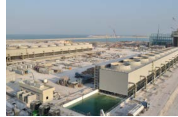
850 MW sea water cooling towers at a combined cycle power plant in Qatar
