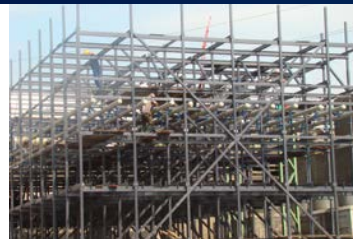
FRP cooling towers – construction phase
