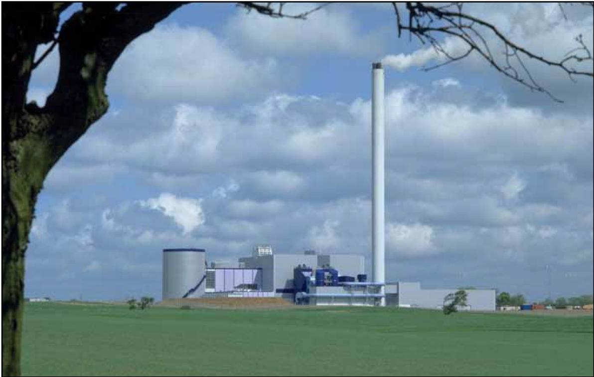
Måbjergværket is the first combined heat and power (CHP) plant in Denmark to use a fuel combination consisting of waste, wood chips, straw and natural gas.
