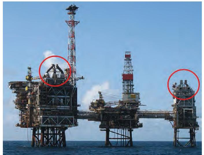
Fig. 1. Typical exhaust system locations (BP Bruce installation, 2011).
