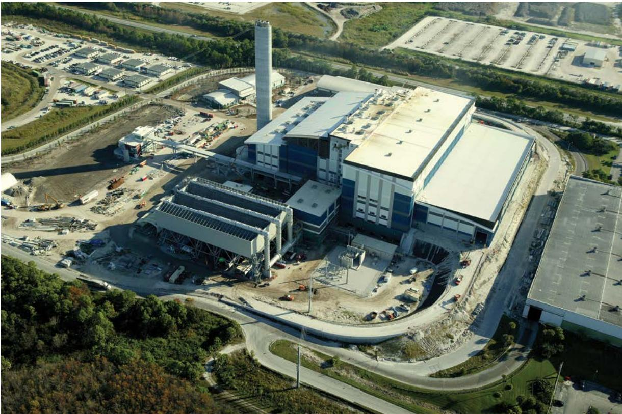
*The state-of-the-art PBREF No. 2 waste-to-energy facility features three B&W boilers and associated emissions control equipment, making it one of the cleanest renewable energy facilities in the United States.*
