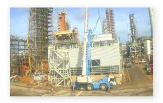
As the 21-day countdown continued, the focus transitioned from construction to the dismantling of the existing wooden tower. Days were dedicated to taking down the existing wooden cooling tower and then preparing the grounds for the installation of the new cooling system.
