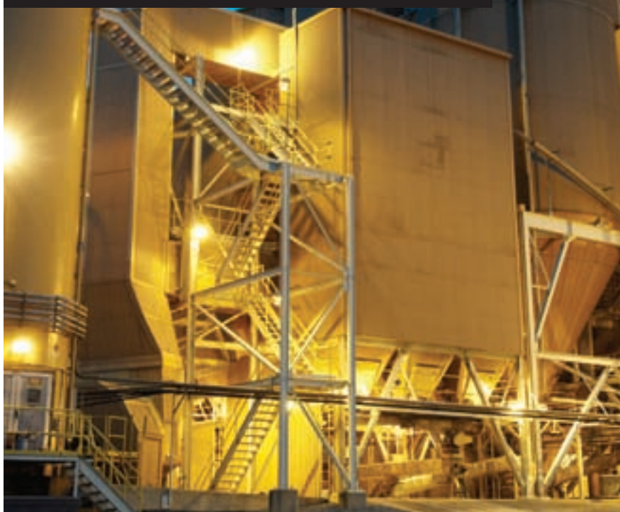
Pulse jet fabric filters for controlling particulate emissions in cement kilns
