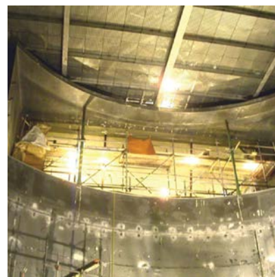
Deposit buildups in the absorber inlet flue are reduced by B&W's patented inlet awning.
