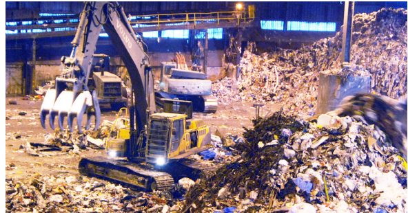
During its first 20-year operating period, PBREF No. 1 processed nearly 16 million tons of municipal solid waste, generated 6.9 billion kilowatts of net electrical output, and recovered more than 664,000 tons of ferrous metals and nearly 63,000 tons of nonferrous metals.
