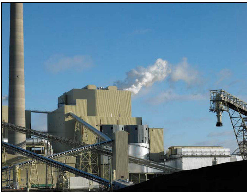
The Weston 4 supercritical boiler utilizes spiral furnace tube technology that provides flexible and reliable operation.
