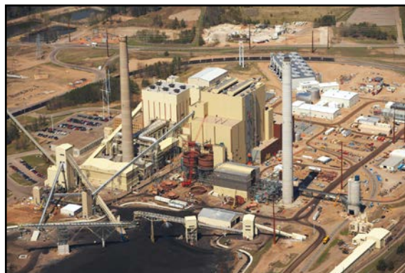
Weston site aerial view during construction.
